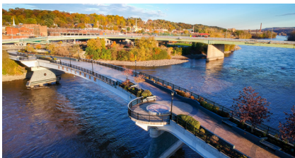
Mohawk Valley Gateway Overlook Pedestrian Bridge Amsterdam, NY
